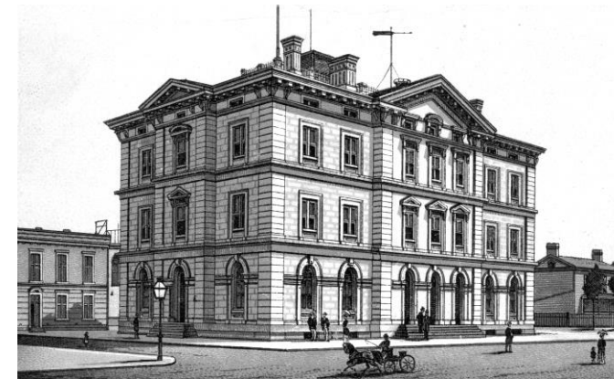
The East Tennessee History Center (Custom House and Post Office, 1885)
